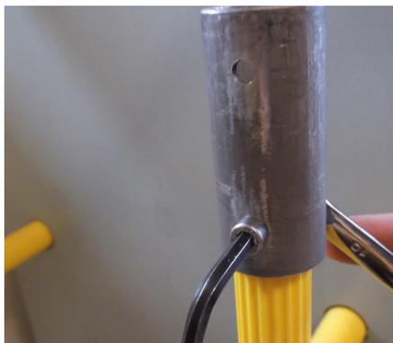
**5.** Square cut the additional length of stringer, pen mark 35mm from the cut end and fit to the rungs. Slide the stringer into the connector upto the pen mark, drill and bolt in place as above.
